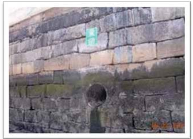
Former CSO Outfall CHE002 now discharges stormwater, only.
