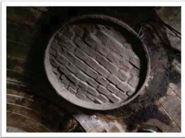
Brick and mortar bulkhead of high outlet overflow in CSO regulator at Outfall CHE002.
