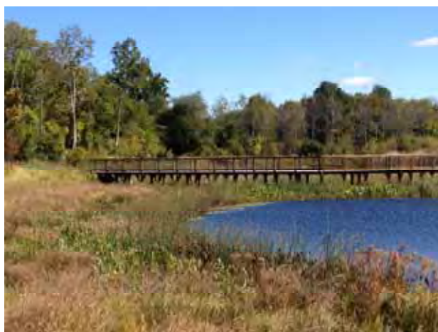
Portion of main wetland basin and boardwalk system
