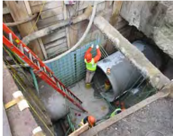
Construction of drain manhole at K and E. 2 nd streets Reserved Channel Contract 3B
