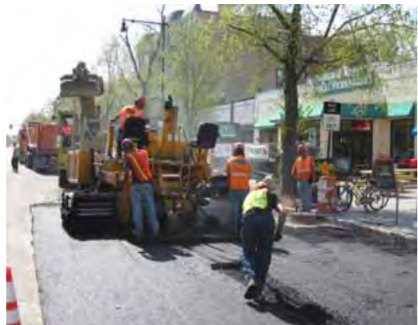
Final pavement restoration following completion of the Brookline Sewer Separation project
