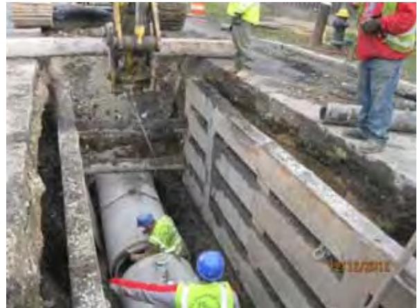
Installation of 36-inch drain on E Street Reserved Channel Sewer Separation Contract 4
