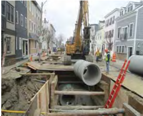
Installation of 48-inch drain on K Street Reserved Channel Contract 3B
