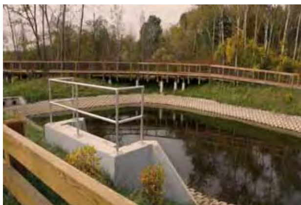
Stormwater outfall and basin "Forebay"
