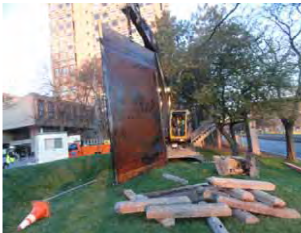
Removal of the overflow plate in Outfall MWR010 completed the Brookline Sewer Separation project
