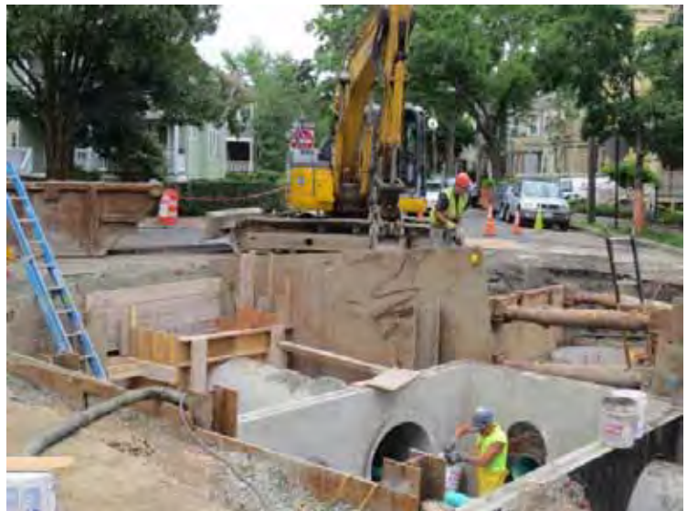
Installation of Drain Vault #1, Vassal Lane and Standish Street, CAM004 Sewer Separation Contract 8A
