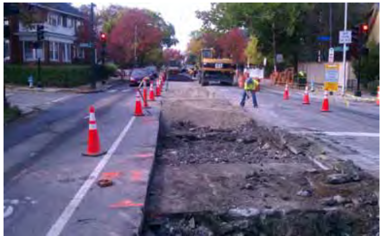
Contract 8B rail track removal along Huron Avenue
