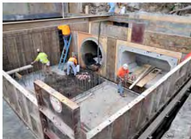
Stormwater Diversion Structure
