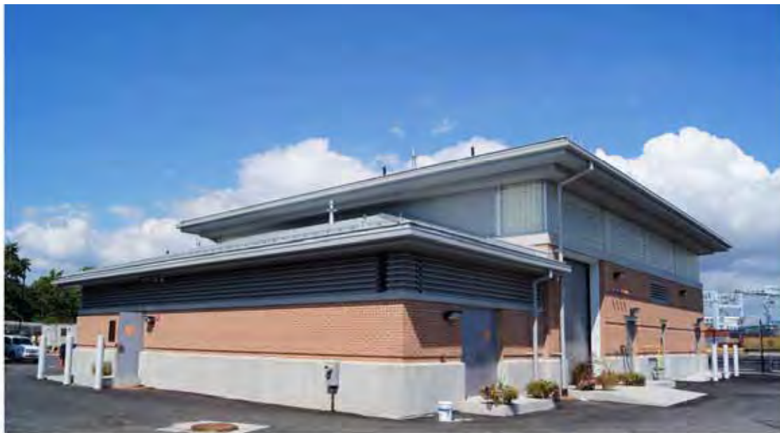
North Dorchester Bay CSO Storage Tunnel Dewatering Pump Station, Conley Terminal, South Boston
