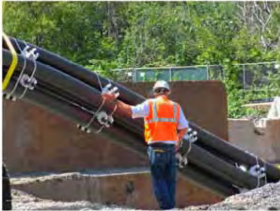
Launching Electric Bundle into Pit
