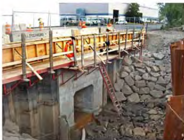
Bridge guard rail and outfall headwall construction on Papas Way
