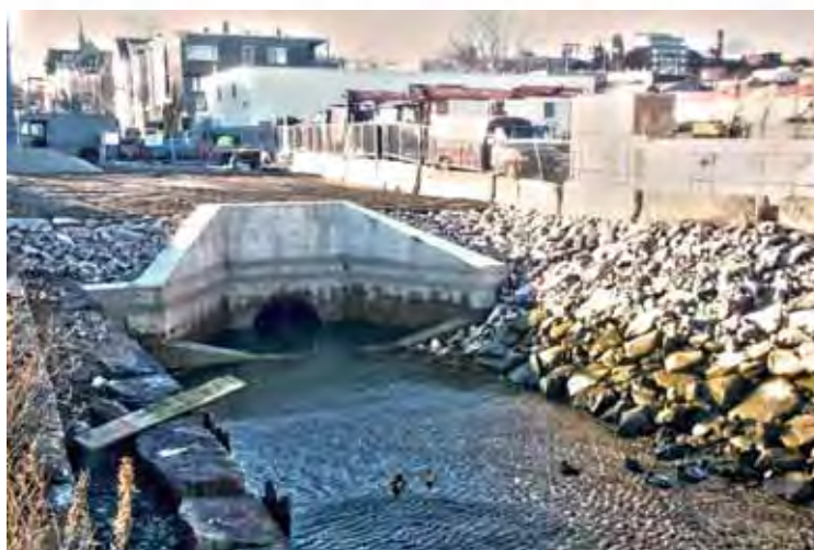
Completed Rehabilitation of Outfall BOS078
