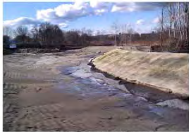
Perimeter Berm at Future Wetland Basin
