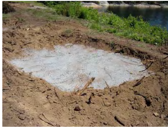
Stump void fill and compaction, prior to final loaming and seeding
