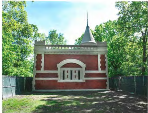
West Siphon Chamber
