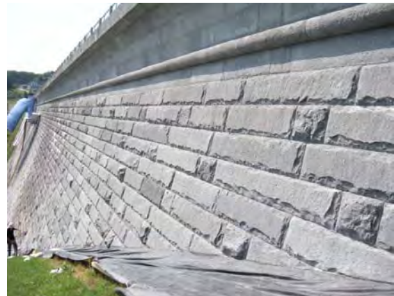
PCB-contaminated efflorescence and mortar
