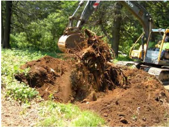
Stump removal from dam
