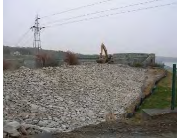
East Berm armored
