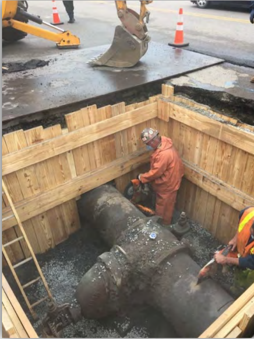
Valve Replacement Section 65
