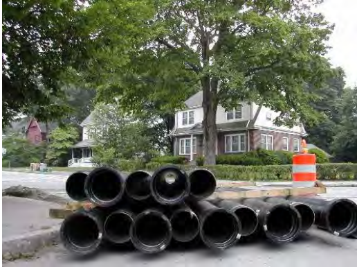
New cement mortar lined mains
