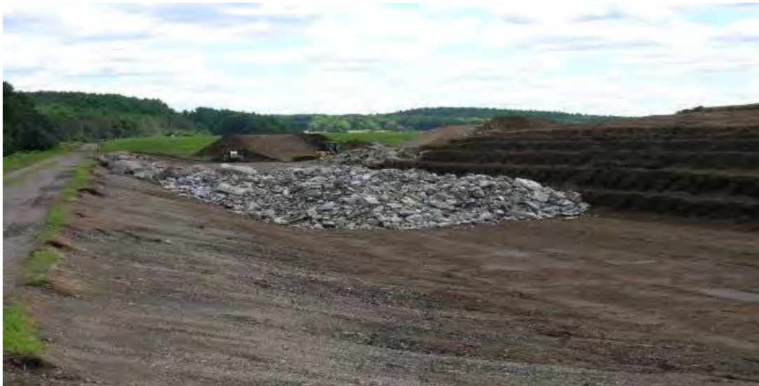
North Dike structural improvements
