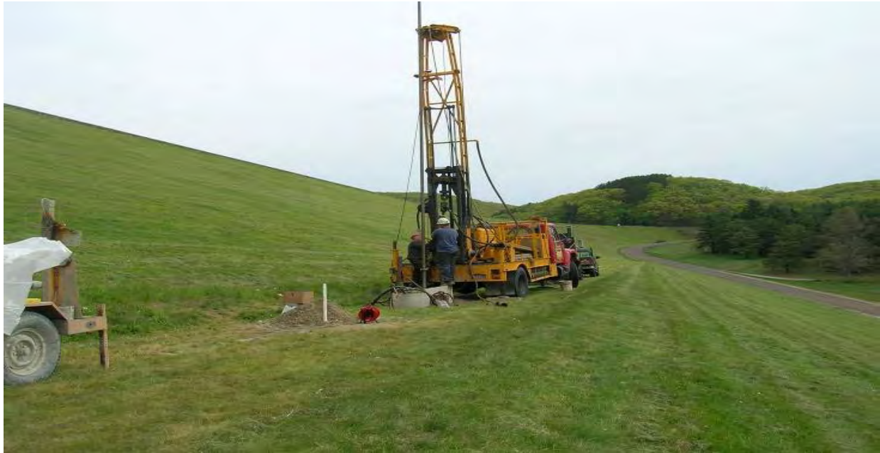
Piezometer Installation at Winsor Dam
