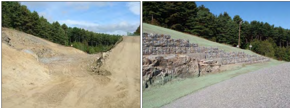
Construction of Auxiliary Spillway (L) and after completion (R)
