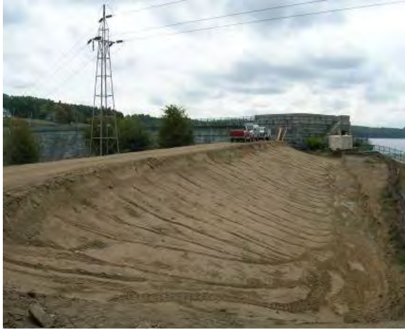
East Berm created along left abutment
