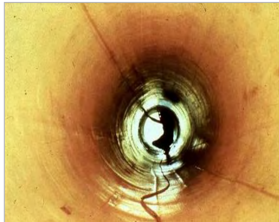
Example of sewer rehabilitated with cured-in-place liner
