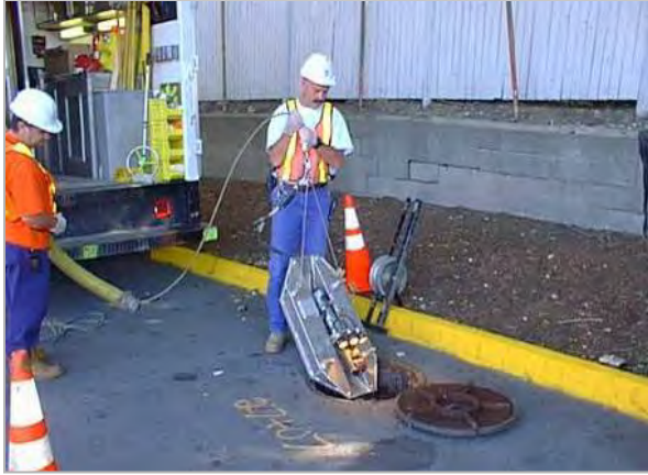
TV Inspection Crew
