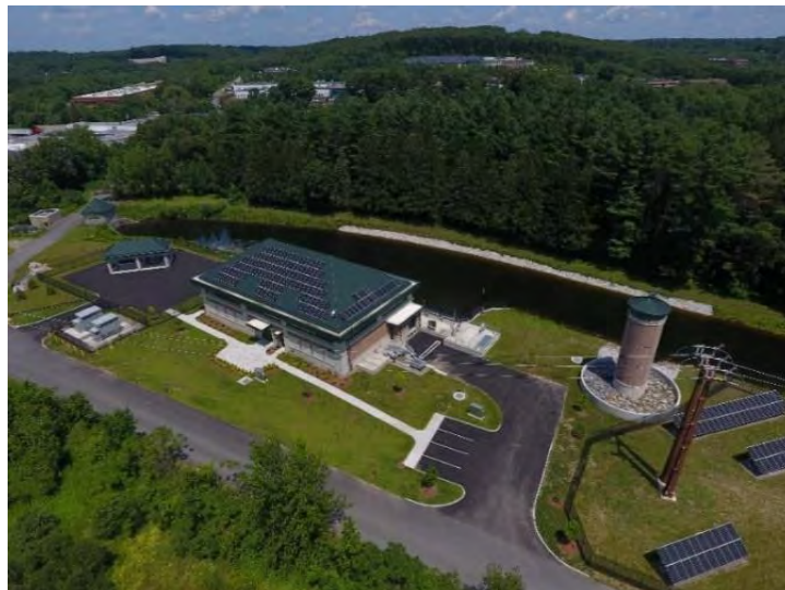
Figure 13: WAPS Geothermal Heat Pump Installation
