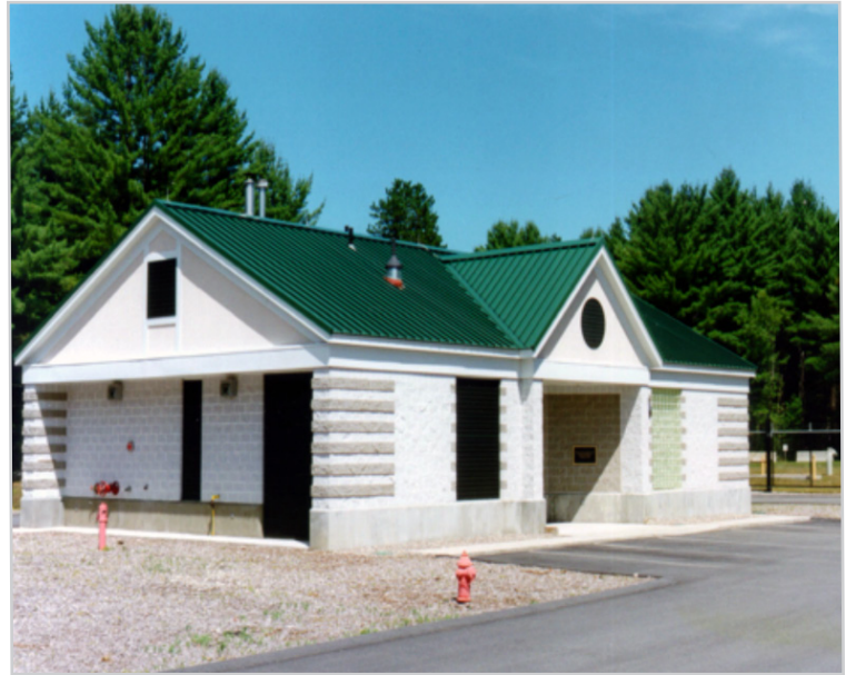
The Quabbin Disinfection Facility in Ware was built in 2000. MWRA is adding UV light water treatment capabilities. The new treatment components will be housed in an addition constructed by Daniel O'Connell's Sons, Inc.
