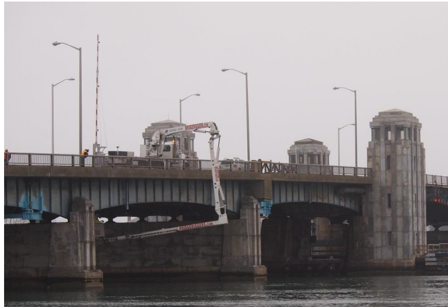
Figure 16 - Accessing Section 56 via Snooper Truck
