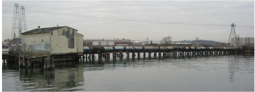
Figure 18 - Historic Railroad Bridge (North)
