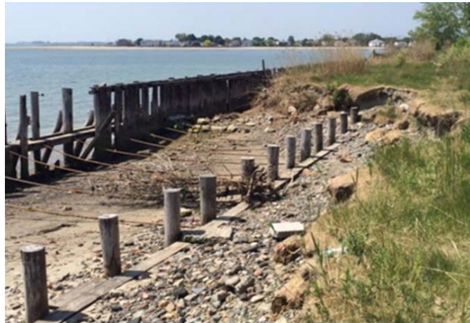
Figure 25 - Lynn Seawall (East)
