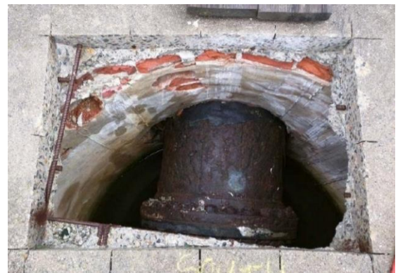
Figure 12 - Inside South Tunnel Shaft
