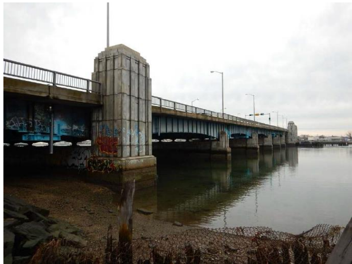
Figure 2- General Edwards Bridge North Elevation
