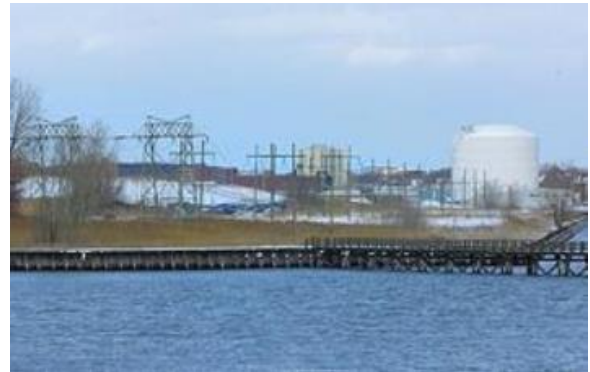
Figure 19 - Historic Power Lines in Harbor Area
