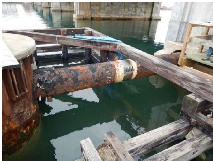
Figure 11 – North Exposed Pipe Section to Tunnel Shaft
