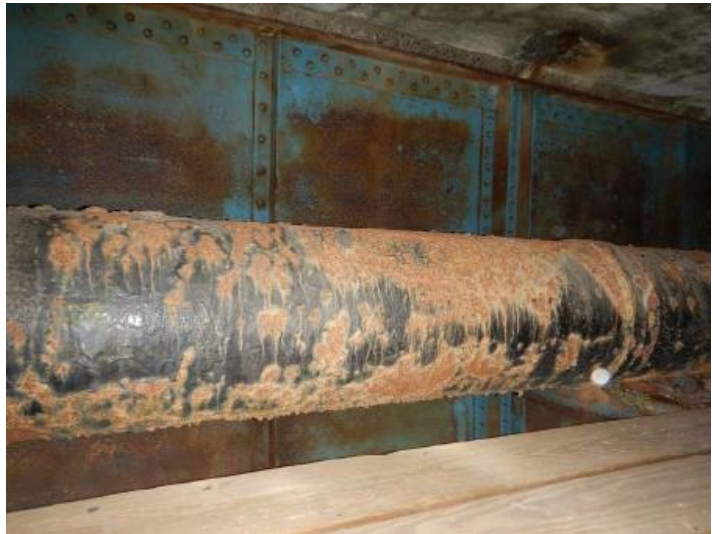
Figure 7 - Typical Exposed Pipe Condition
