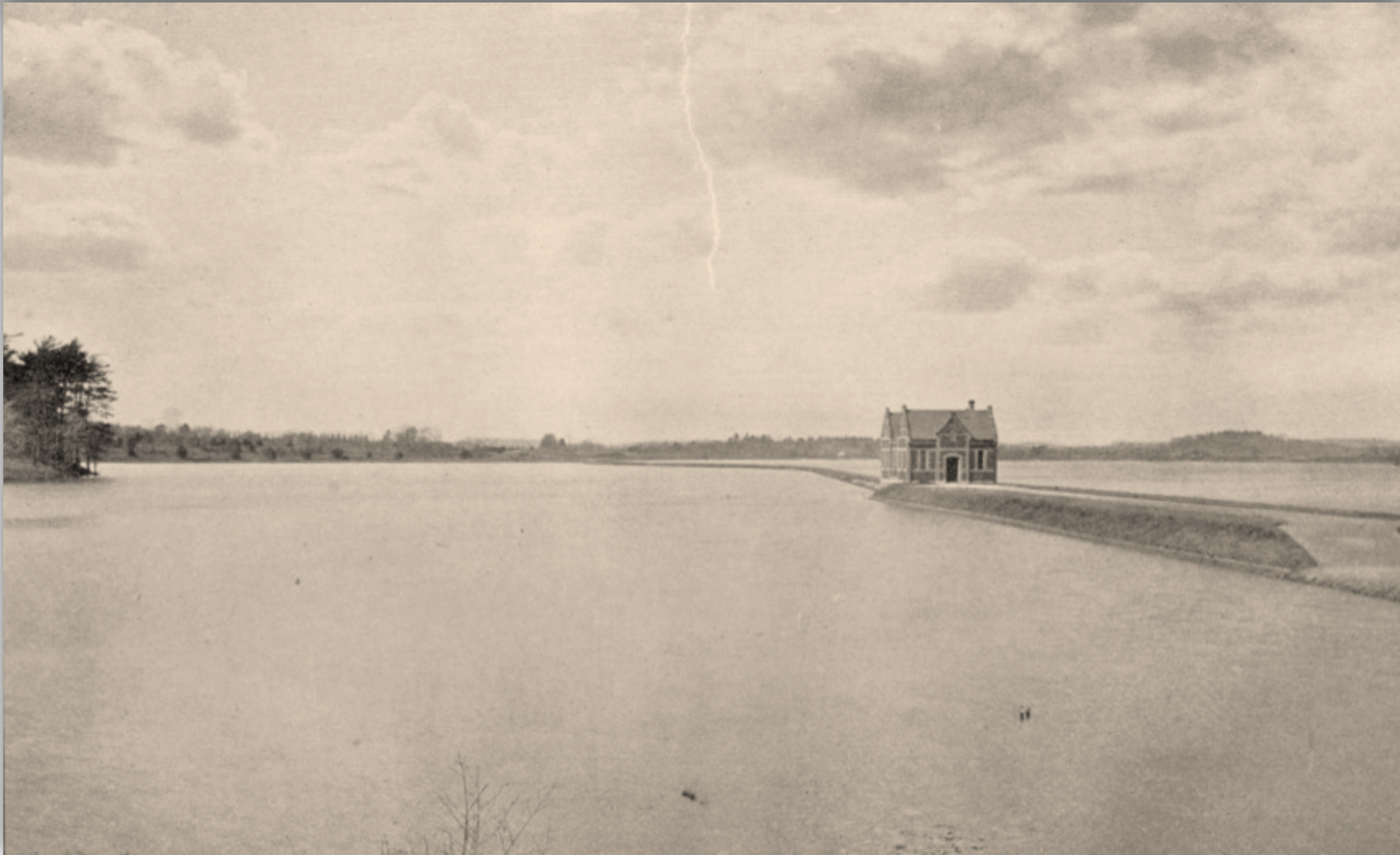
The Farm Pond Gatehouse in Framingham, the aqueduct literally crossed the pond
