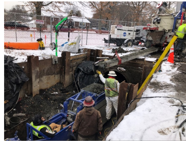
WASM 3 Pipeline Rehabilitation
