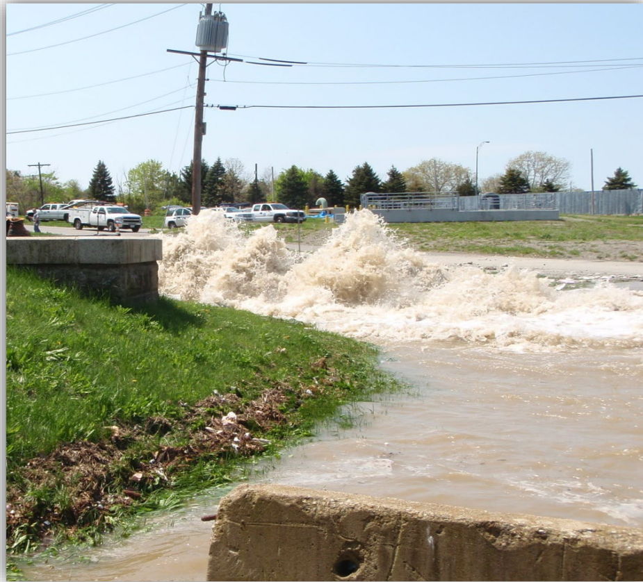
250 MGD flow at Shaft 5 break....
