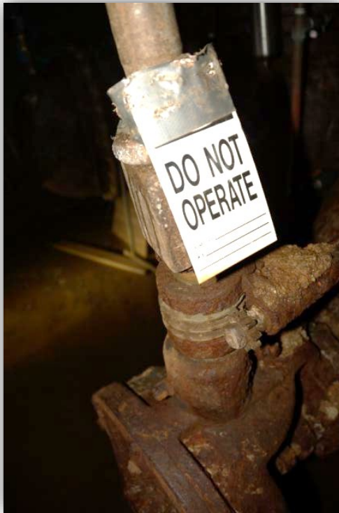
Shaft 8 PRV Chamber
