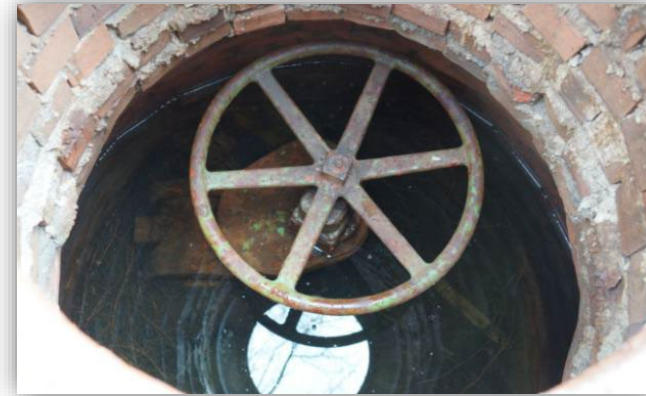
Shaft 7C connection to Section 58
