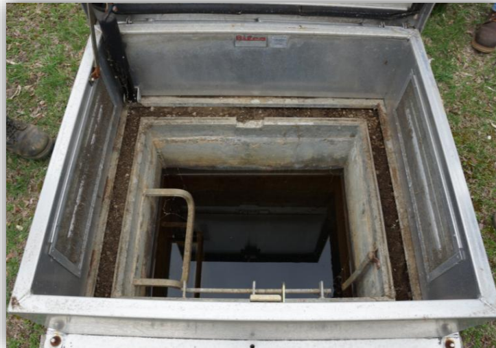
Chamber at Shaft 7C
