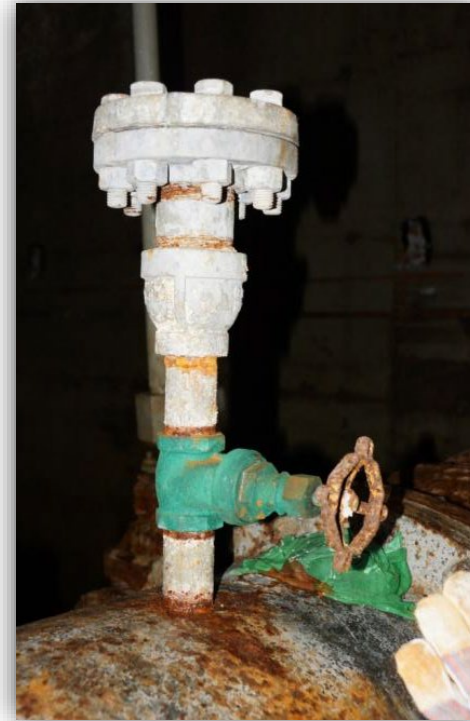
Shaft 8 PRV Chamber
