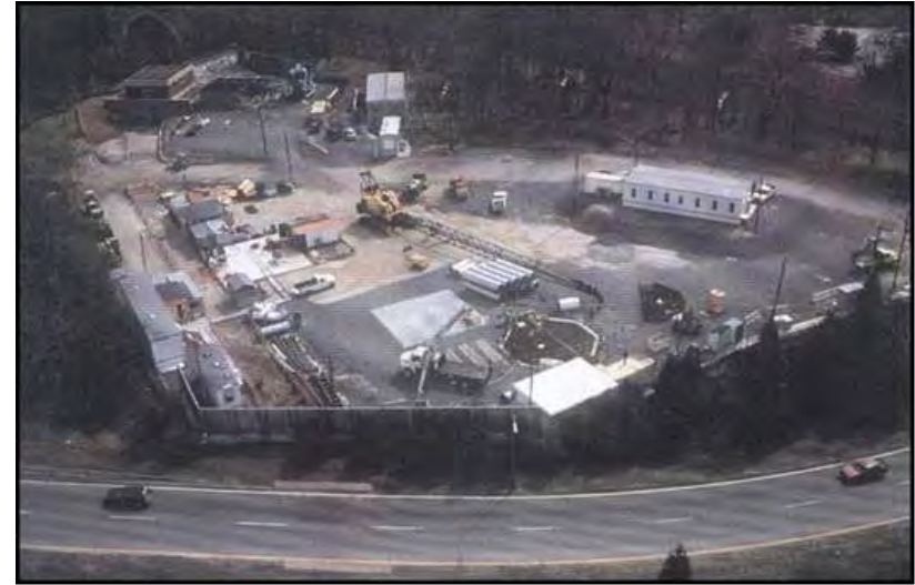
Shaft Site During Construction
