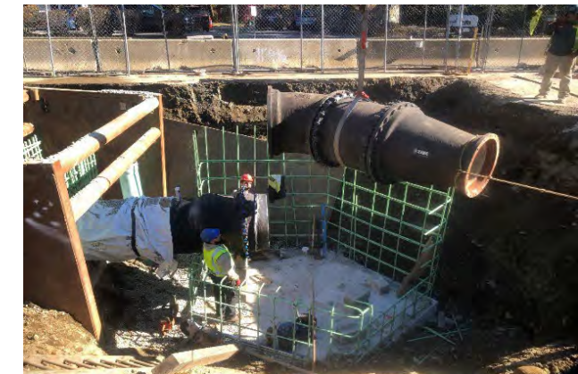
36" pipe & thrust block @ Lexington St & Totten Pond Rd
