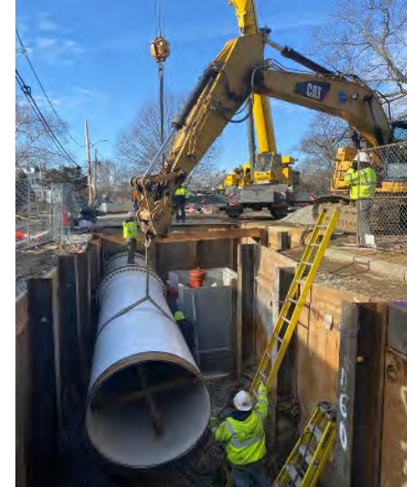
WASM 3 – pipe replacement
