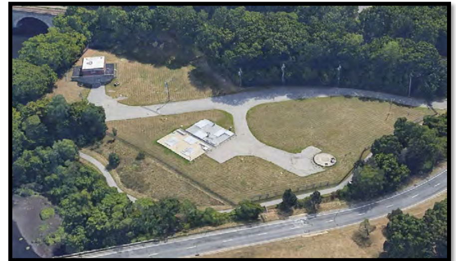
Shaft Site After Construction
