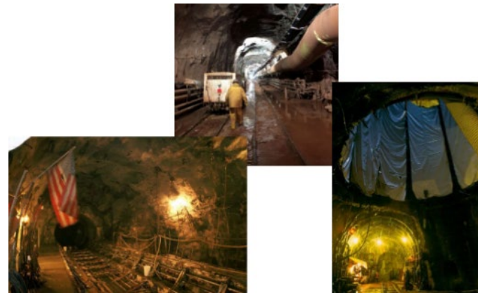
Example of tunnel boring activities
