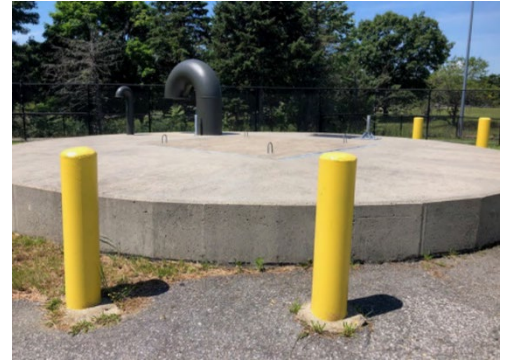
Example of final conditions of a shaft
