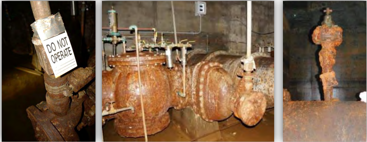
Figure 1 – Condition of Some Existing Tunnel System Valves
