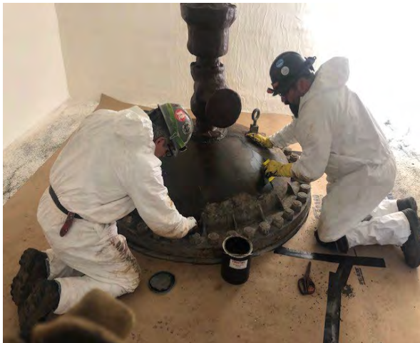
Figure 3 – Protective coating for top of shaft appurtenances
