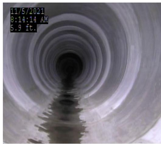
*WASM 3 Cleaned and Lined Piping*
