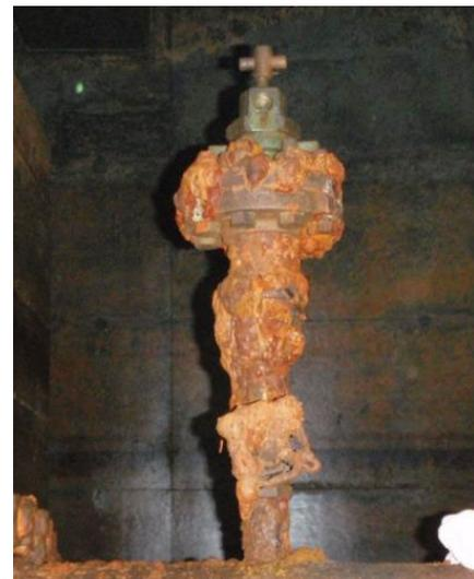
Corroded air valve at Shaft 9A
