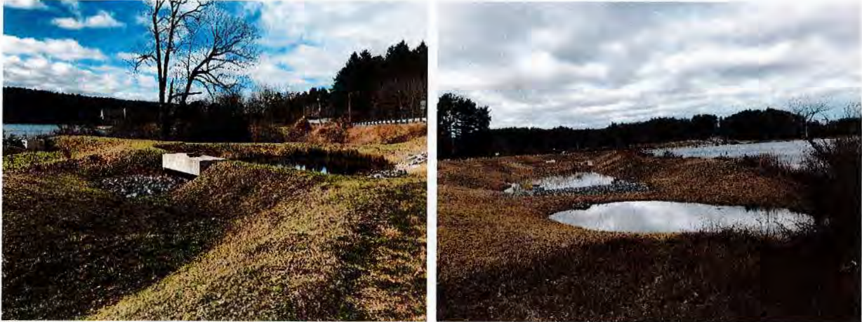
Wachusett Reservoir Direct Discharge Elimination System basins
