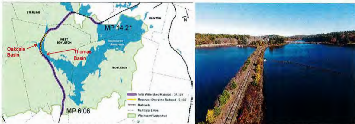
PanAm RR Track within Wachusett Reservoir watershed (L) and causeway (R)
