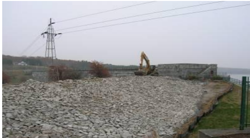
Wachusett spillway east berm construction
