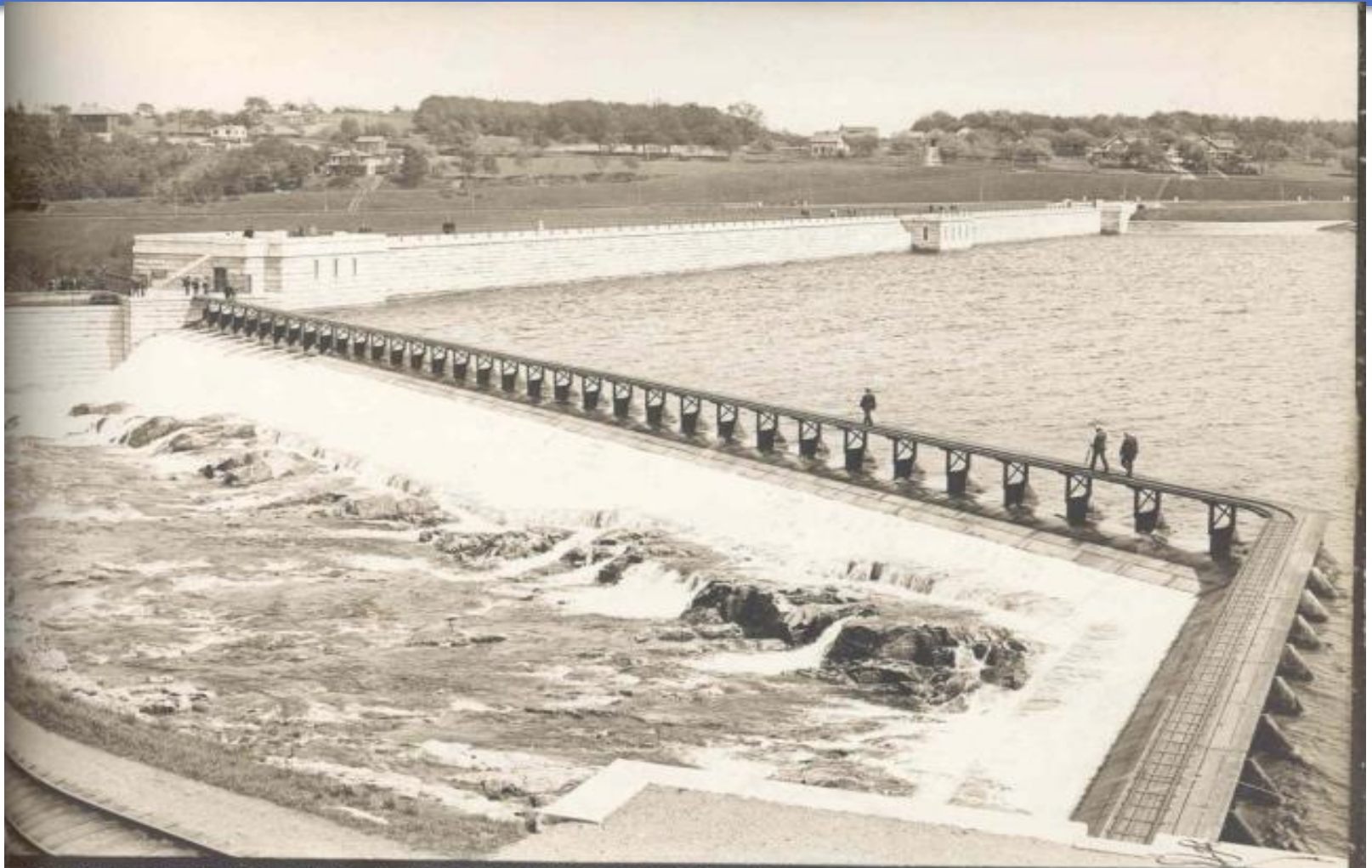
WACHUSETT DAM, CLINTON, FROM THE WEST. MAY 27, '08.
