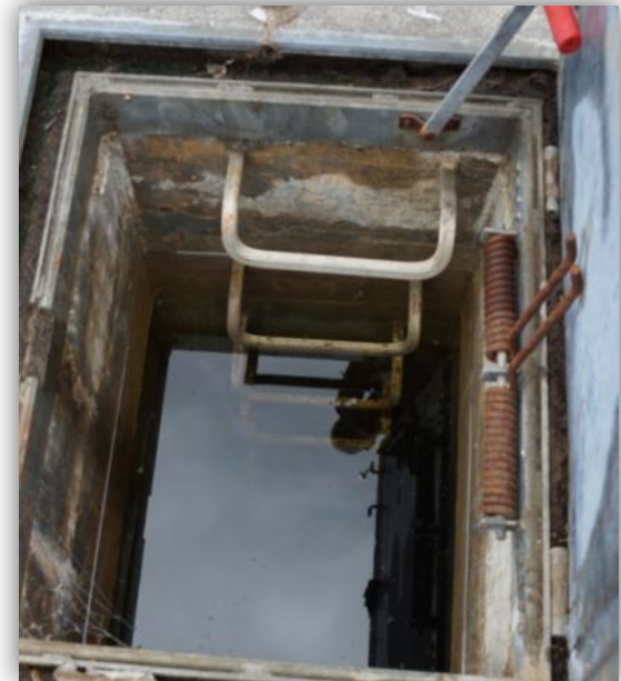
Chamber at Shaft 7D
