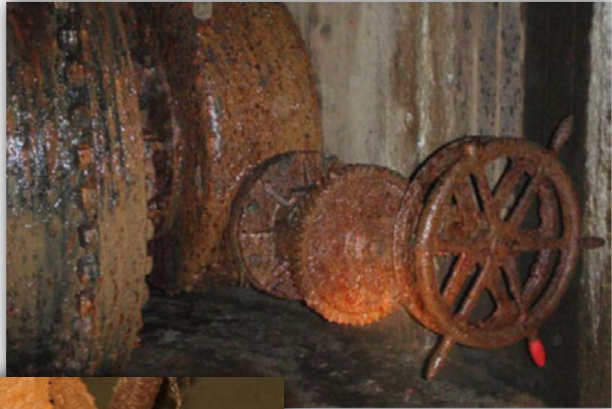
Cone Valve at Shaft 7B
