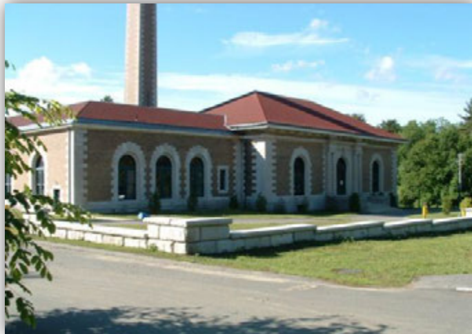
Gillis Pump Station (1899)
