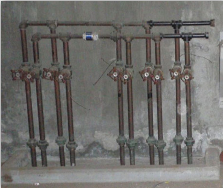
Valve control piping still present in both shaft buildings
