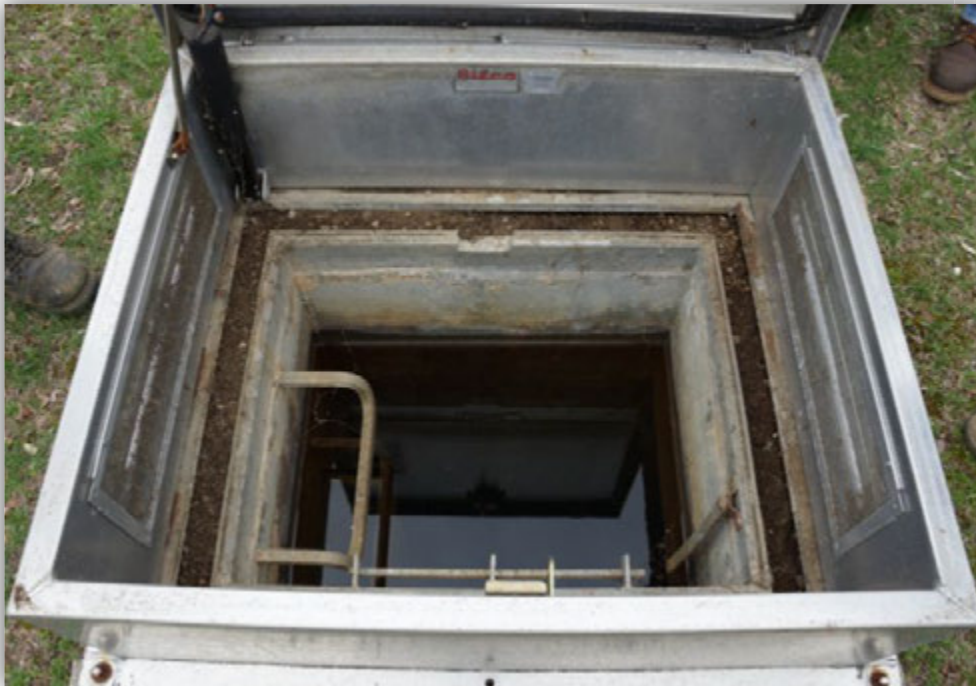
Chamber at Shaft 7C
