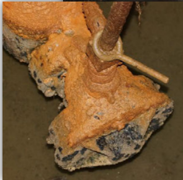
Gear box on valve at Shaft 8
