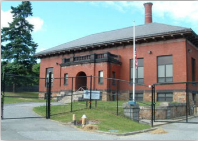
Brattle Court Pump Station (1907)
