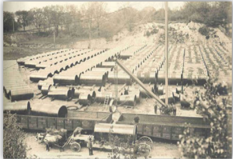
WASM 1 and 2 Pipe Yard (1915)
