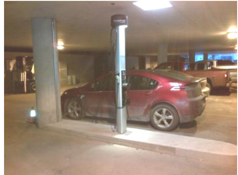
Center island allows 4 cars to charge without moving a vehicle
