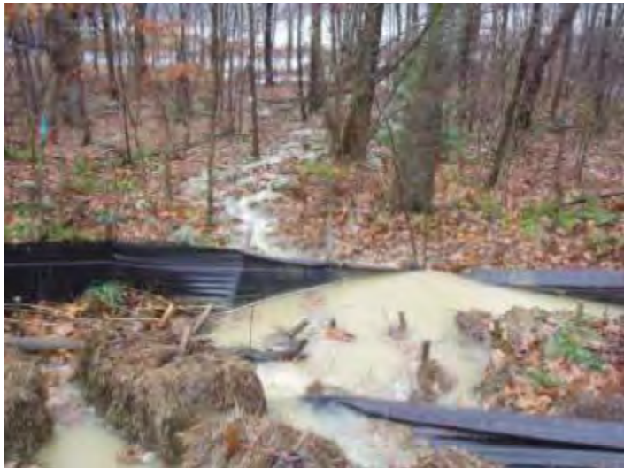
Overwhelmed erosion controls with sediments flowing through wetland to Moulton Pond, November 2008.
