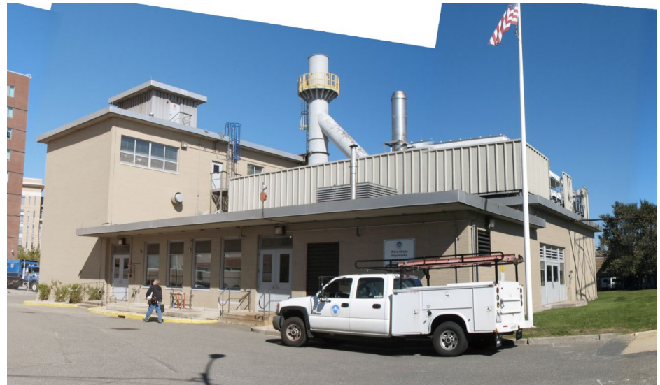
Existing Ward Street Headworks
