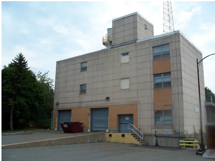
Existing Columbus Park Headworks
