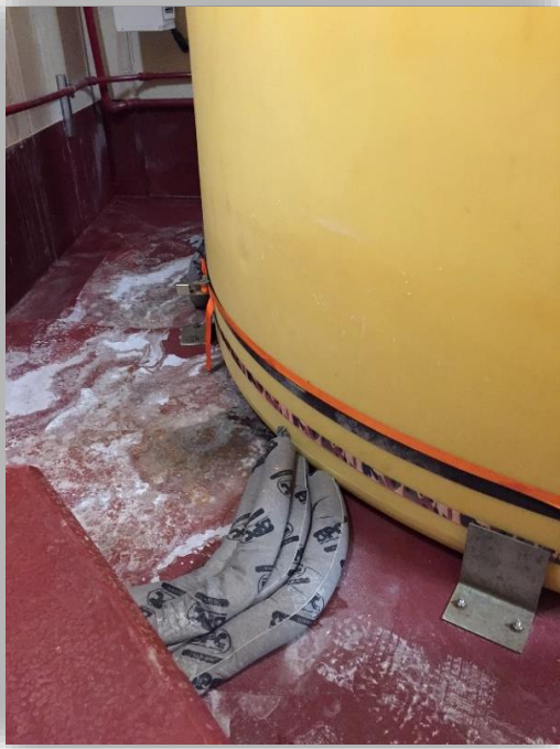
Replacement of Leaking Chemical Tanks
