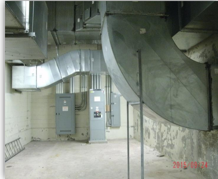
Relocation of Electrical Room
