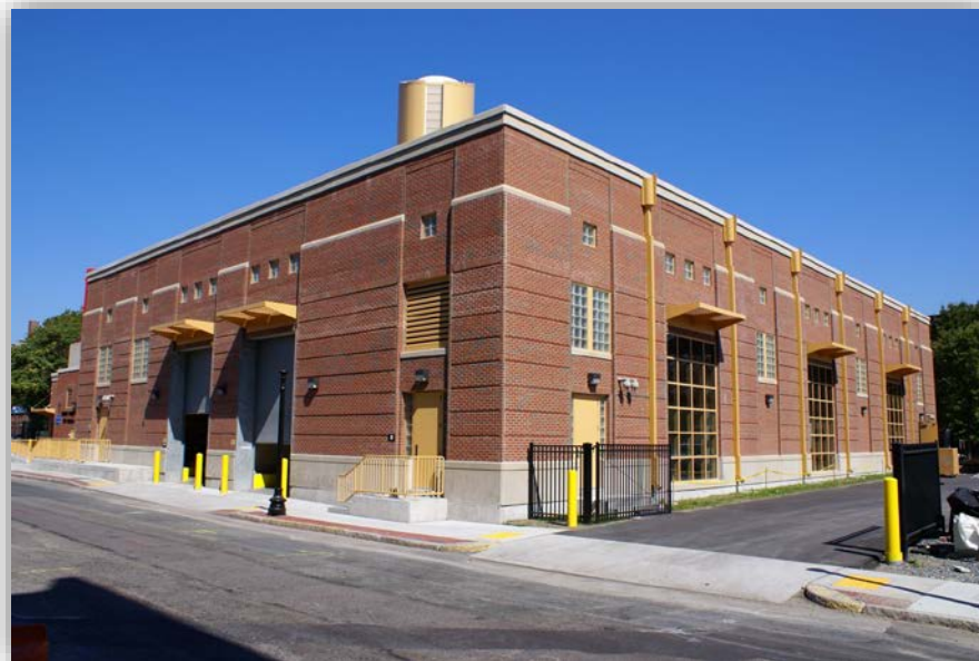
Union Park detention/treatment facility
