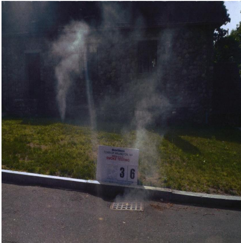
Catch Basin Direct Connection to Sewer
