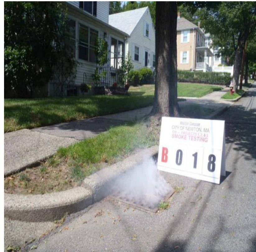
Catch Basin Direct Connection to Sewer
