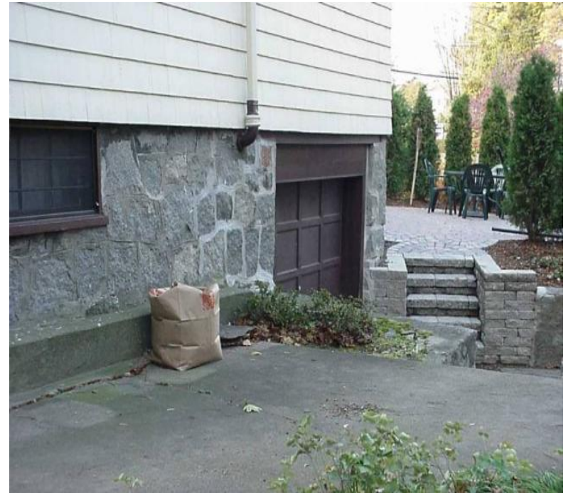
Downspout Direct Connection to Sewer
