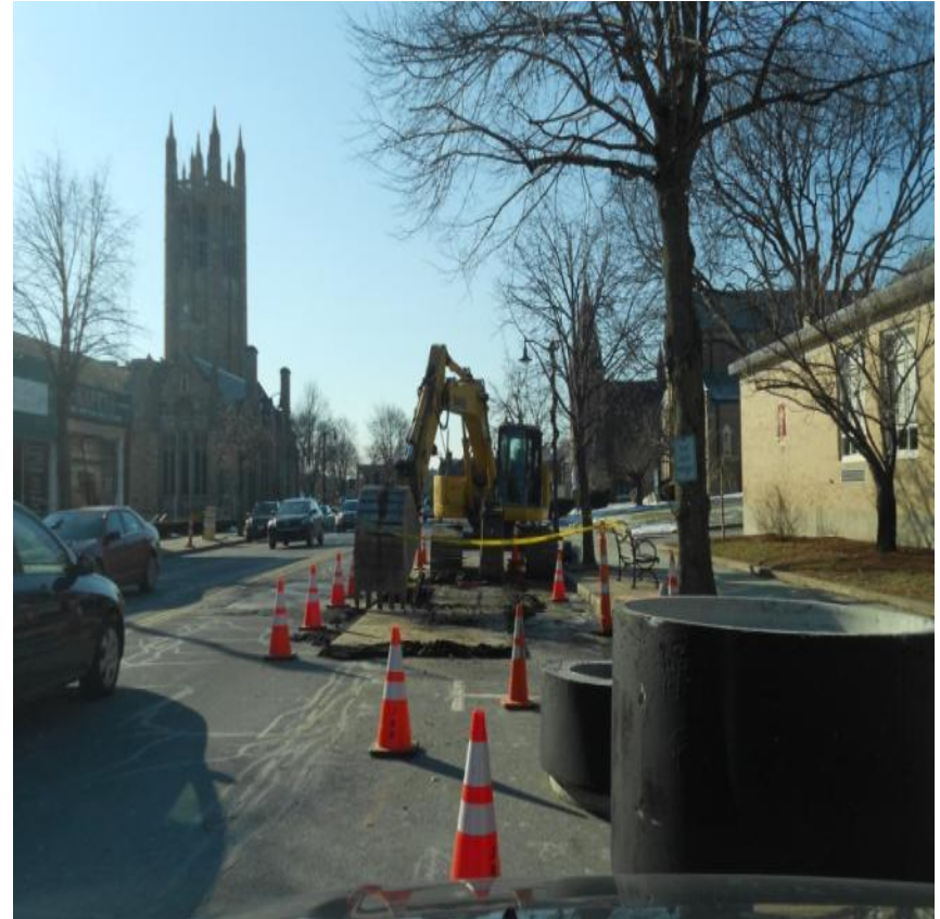
Sewer Spot Repair and New Manhole
