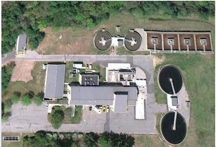
The MFN (Mansfield-Foxboro-Norton) Regional Wastewater Facility in Norton is managed by a regional entity that took six years to create.
