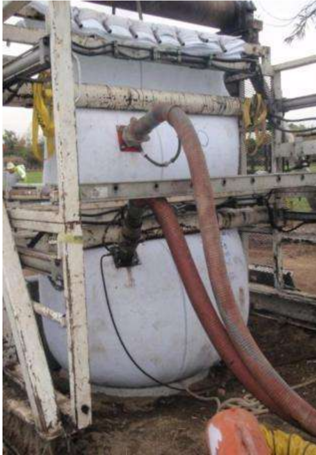
CIPP air/steam process
