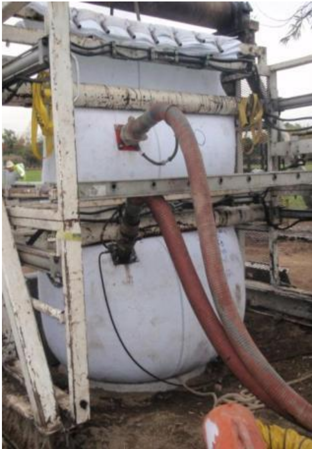
CIPP air/steam process
