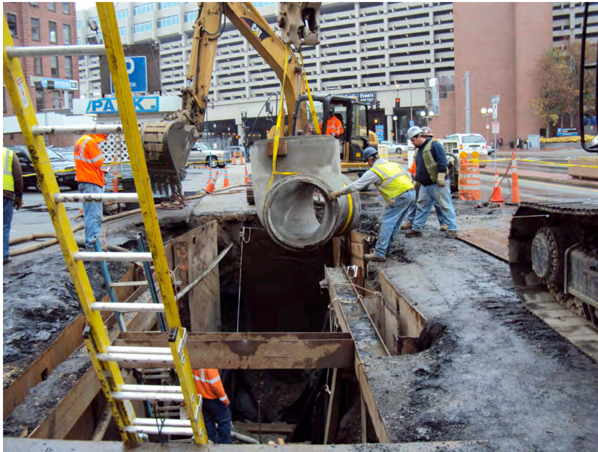
Installation of 42" storm drain on Merrimac Street
