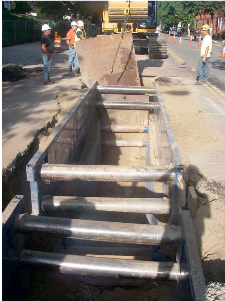
Installation of force main in East Broadway.
