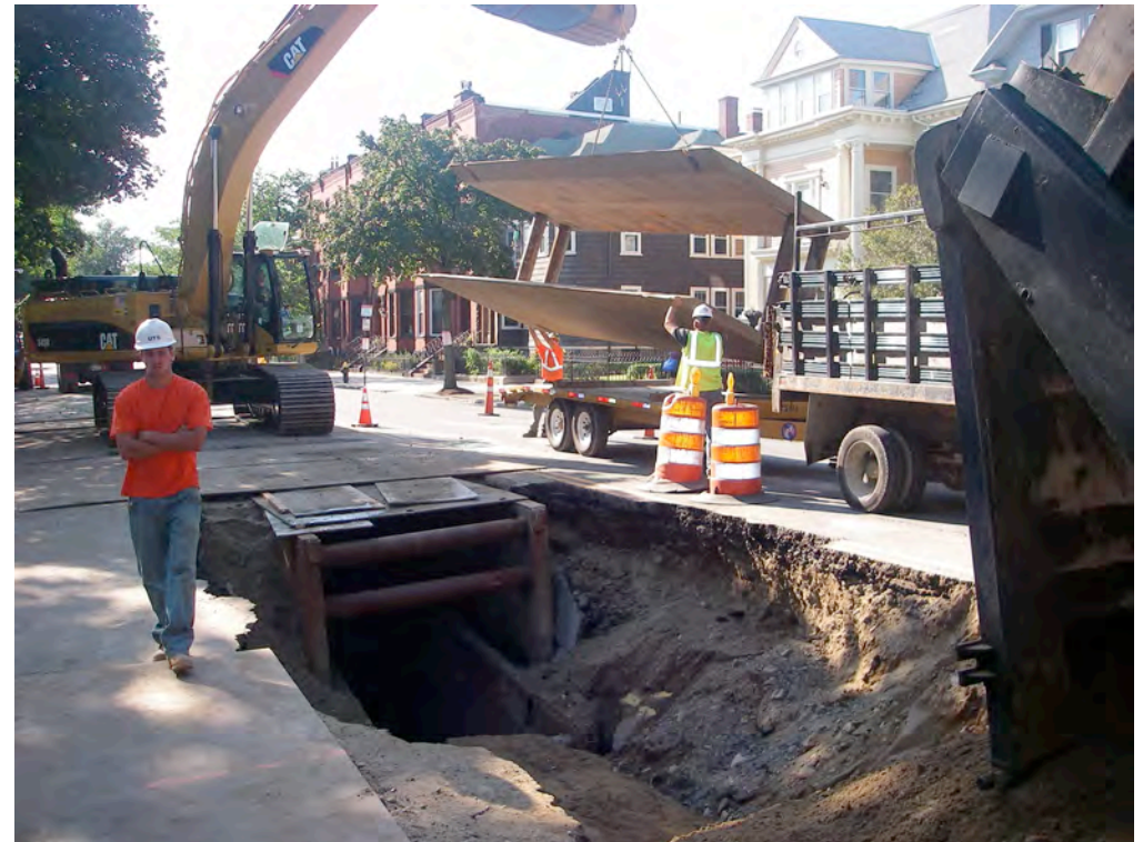
Installation of force main in East Broadway.
