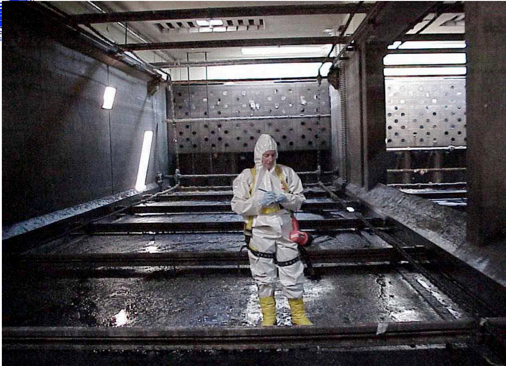
Interior of Primary Clarifier-Battery A
