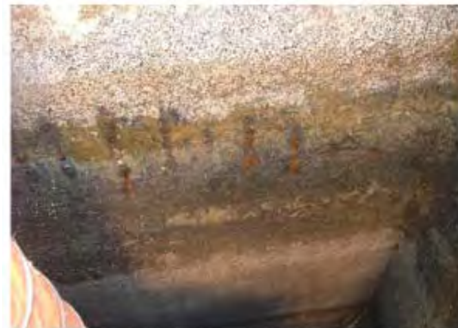
4) GTO Wet Well #4 Wall
