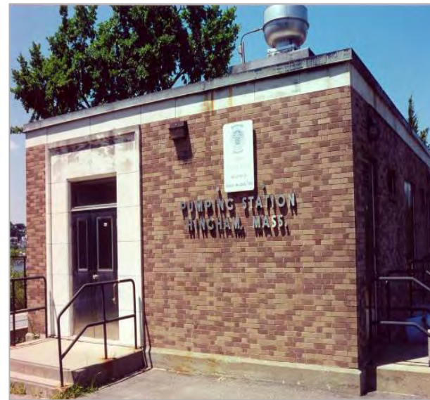
Hingham Pump Station (1992)
