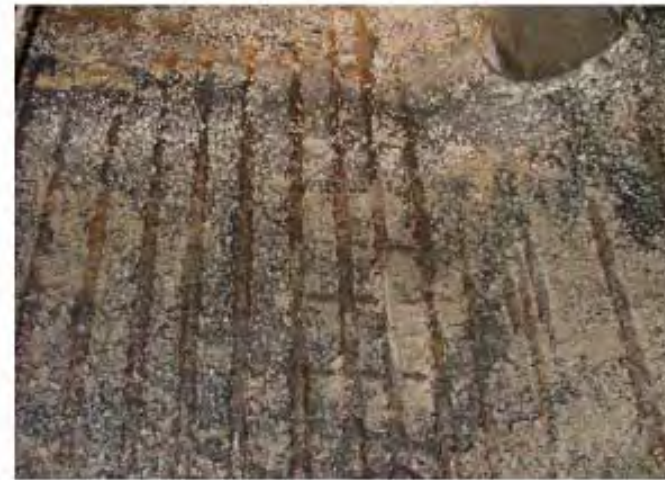
2) GTO WET WELL #3 Wall
