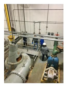
Lead paint peeling  $\rightarrow$  that, PCBs and asbestos will all need to be remediated as part of the facility rehabilitation.
