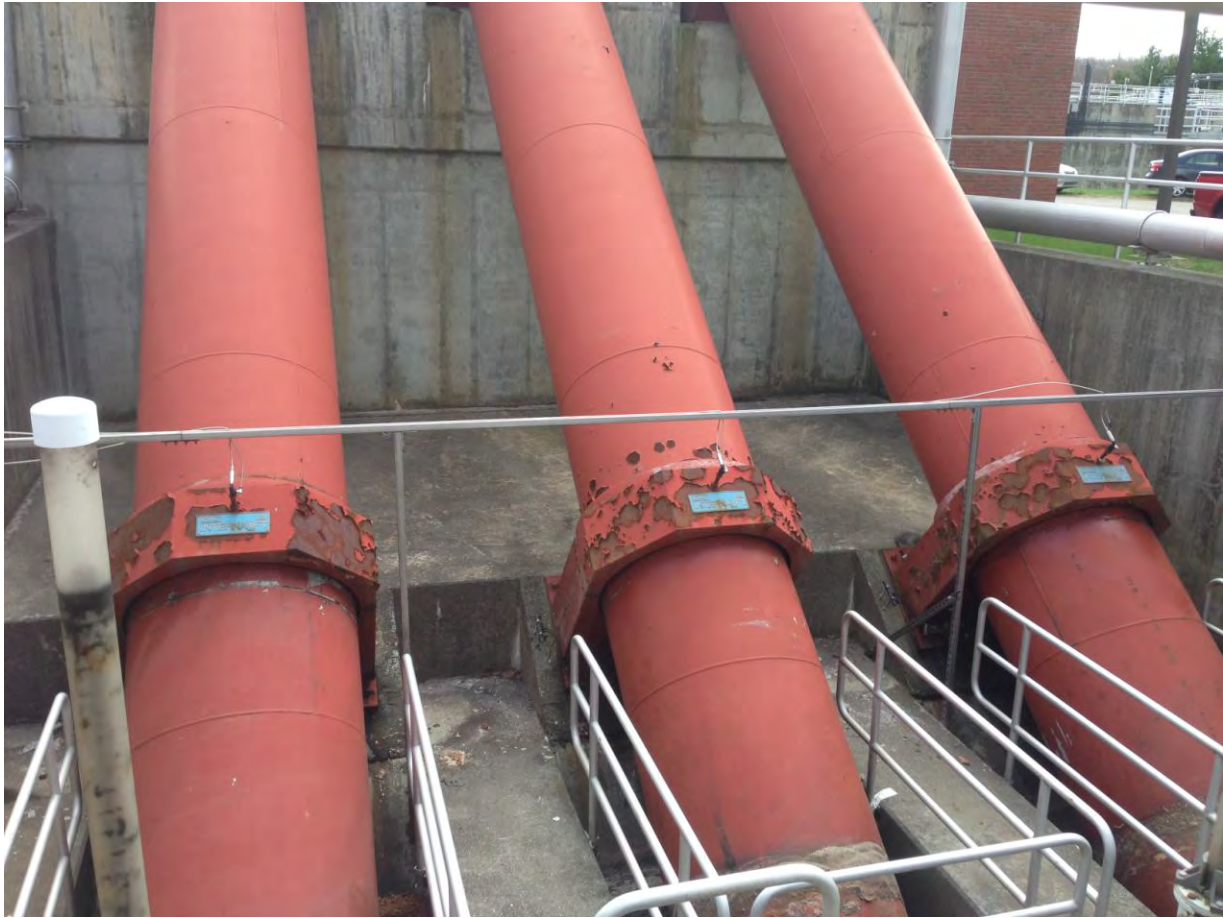
(Influent screw-lift pumps. These remain about a third full of water even when off)
