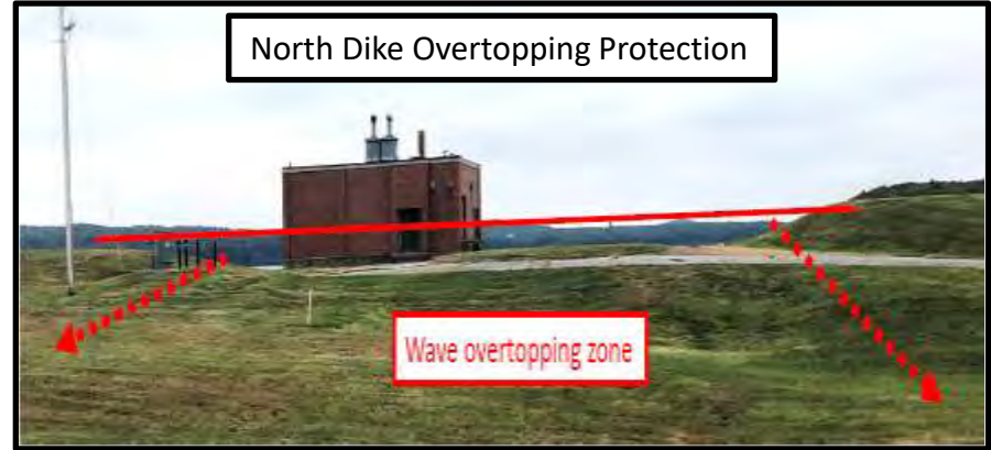
Foss Dam Overtopping Protection
