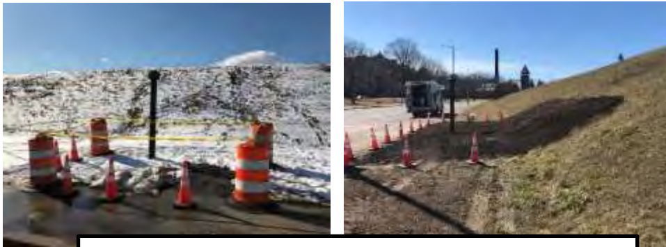
Chestnut Hill Dam Seepage Repair (added by Amendment)
