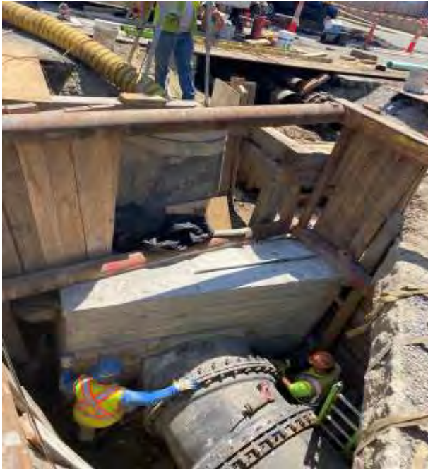
New Concrete Headwall
