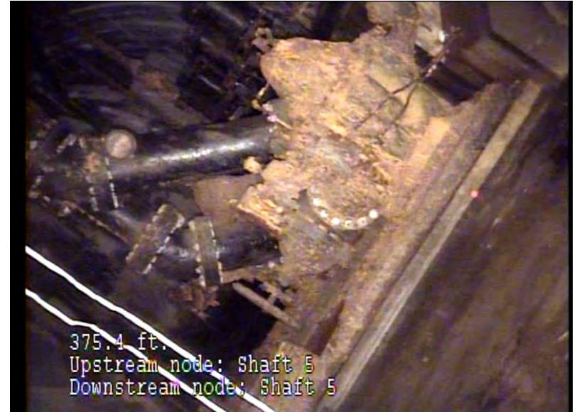
Underground pump room (abandoned with fill)
