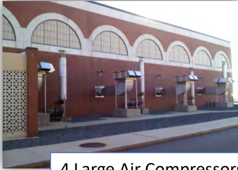
4 Large Air Compressors (2 @ 2,000hp, 2 @ 2500 hp)
