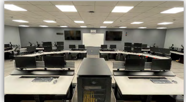
New Control Room
