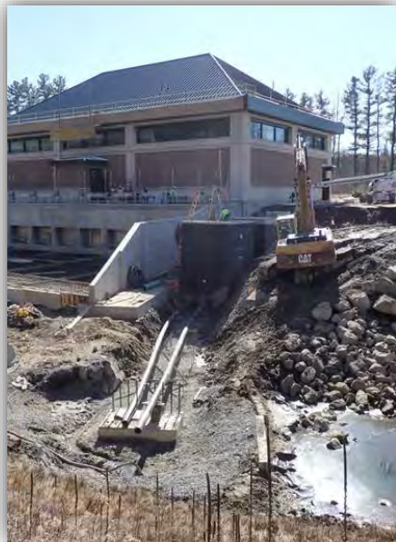
Wachusett Aqueduct Pump Station Geothermal Heat Pump During Construction
