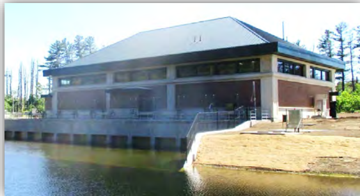
Wachusett Aqueduct Pump Station After Construction
