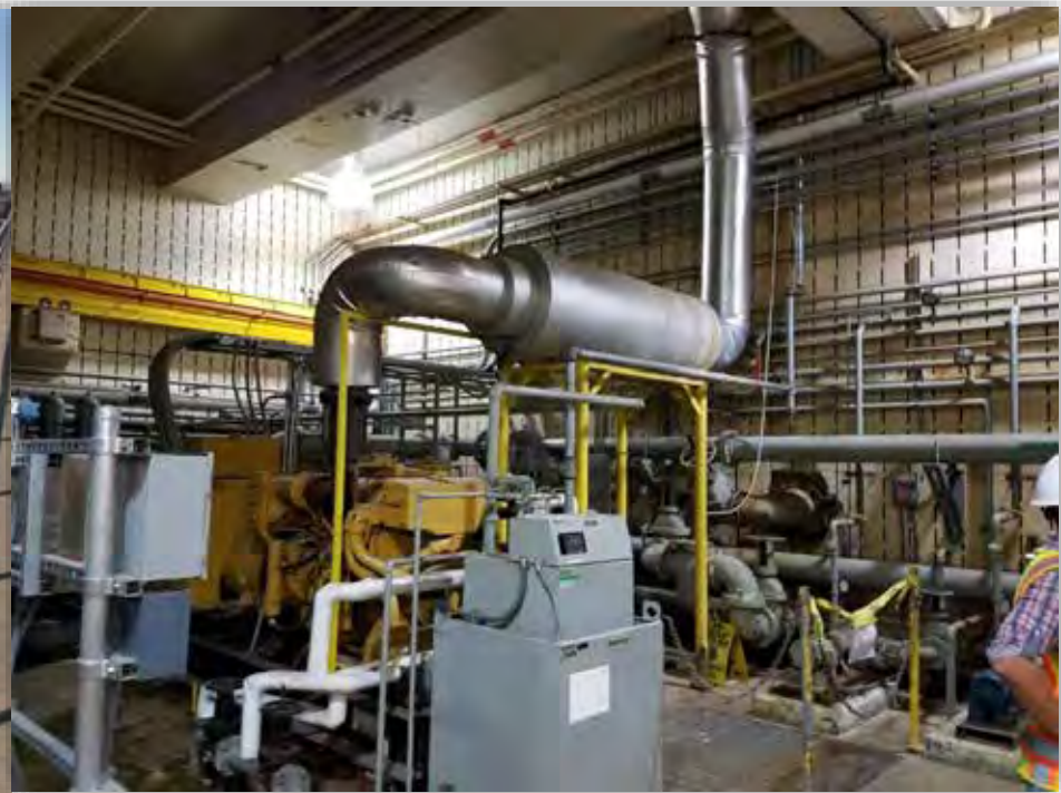
Prison Point Rehab Construction
