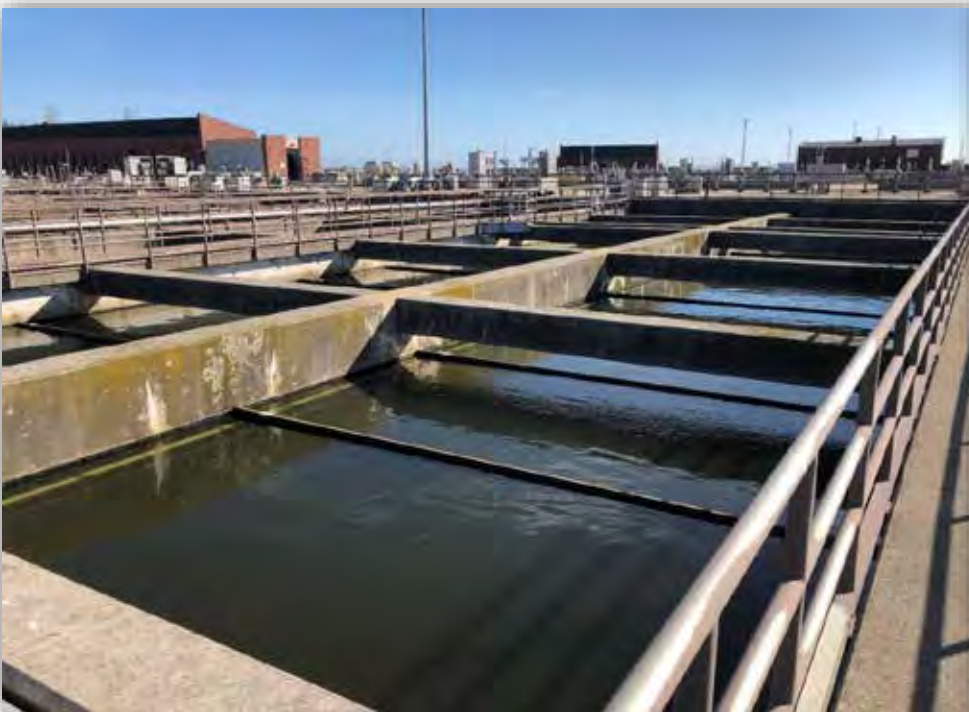
Clarifier Rehab Phase 2 Construction
