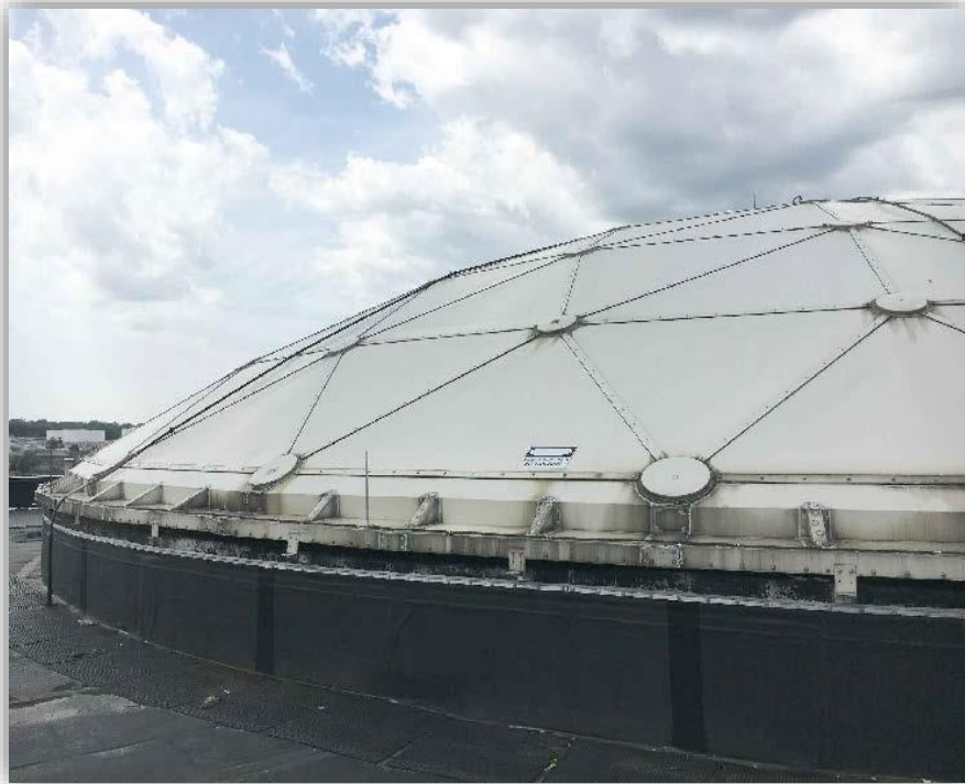
Sludge Tank Roof Cover (braces under roof cover)
