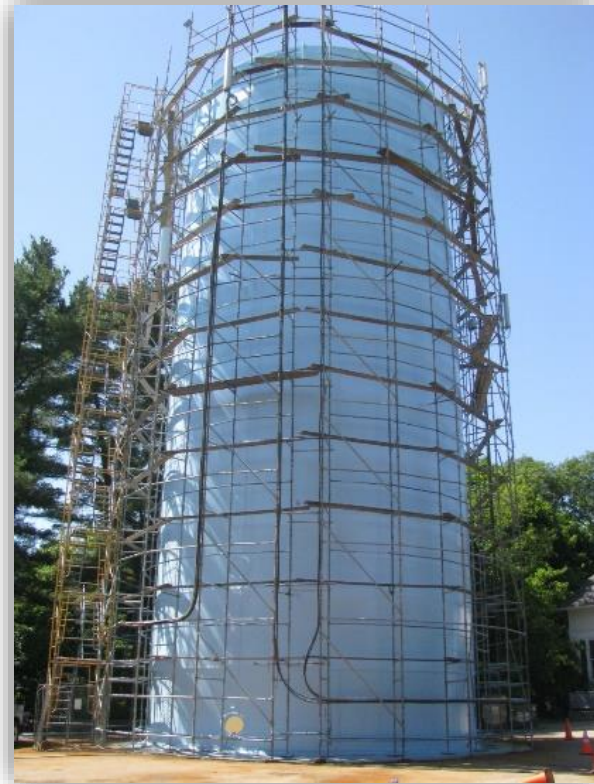
Water Storage Tank Rehabilitation
