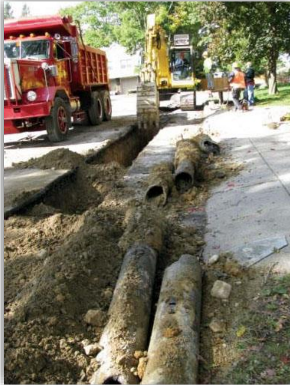
Water Main Replacement Construction
