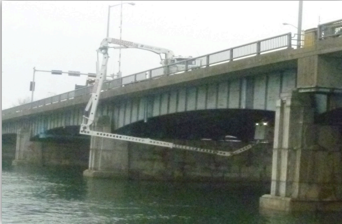
General Edwards Bridge Water Main Inspection
