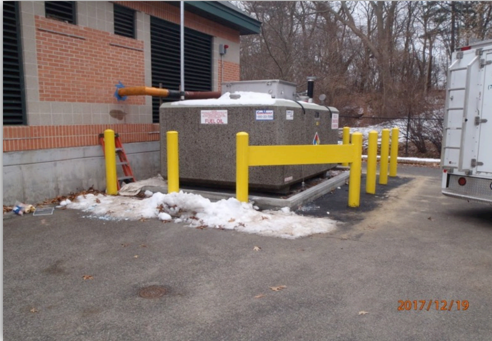
Completed Quincy Fuel Tank Replacement
