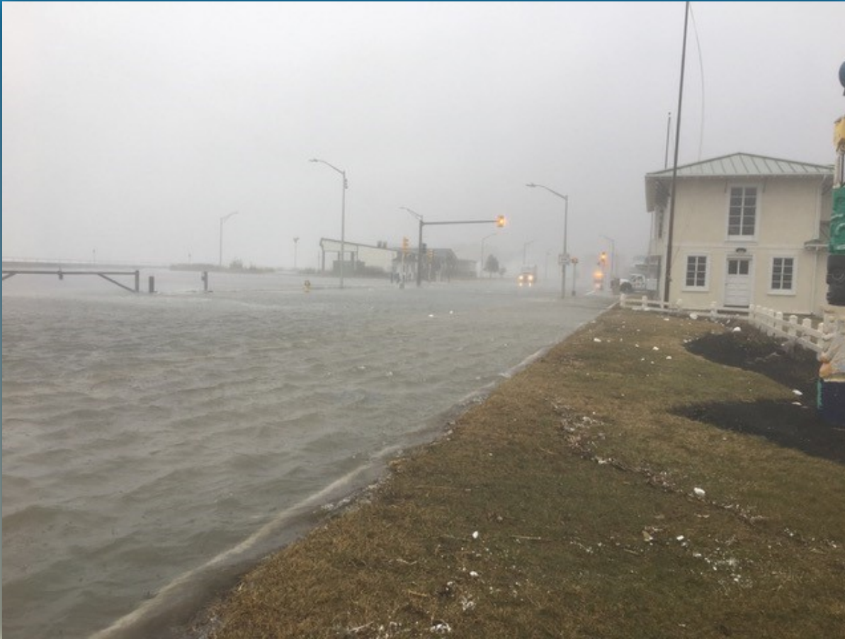
Nantasket Avenue in front of DCR complex; damage to Hull Shore Drive
