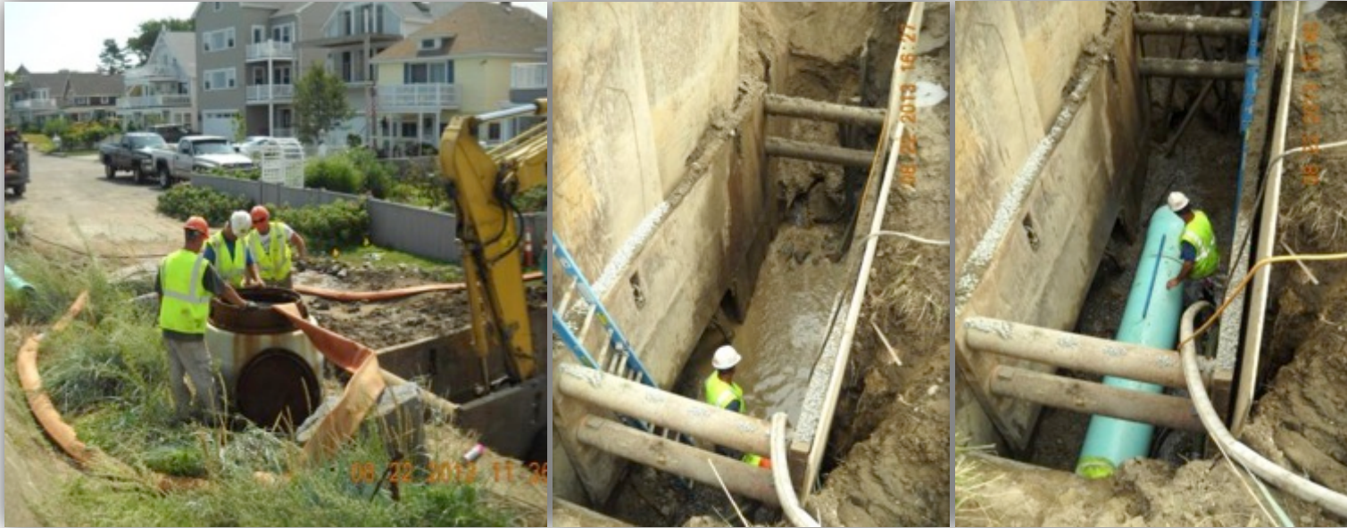
Quincy sewer repair at Salt Marsh
