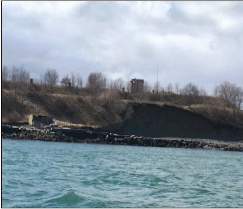
Looking south, showing continued damage to historic seawall and outer earthworks of Fort Warren
