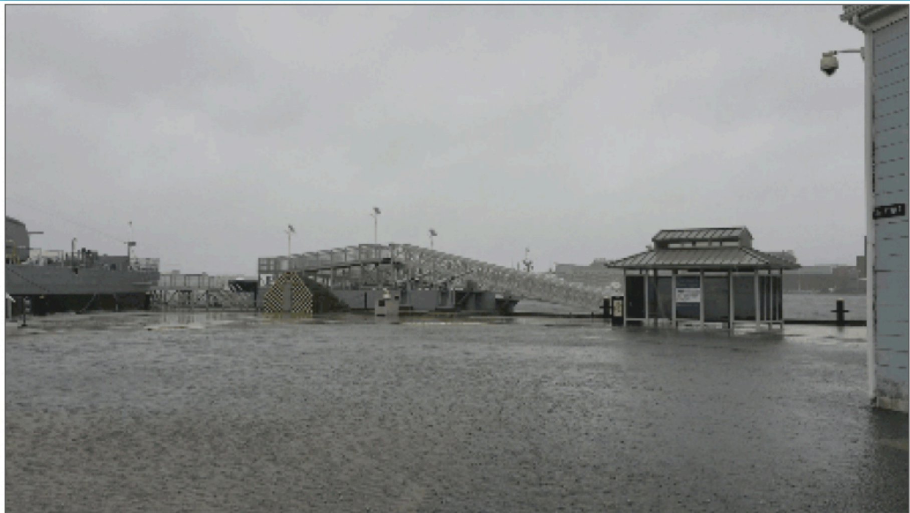
Pier One was flooded from overtopping of seawall
