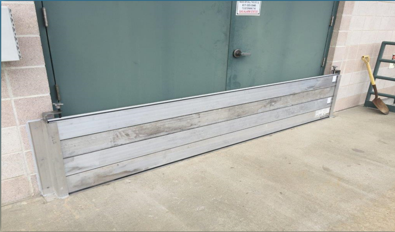
Stop logs installed to keep facilities from flooding
