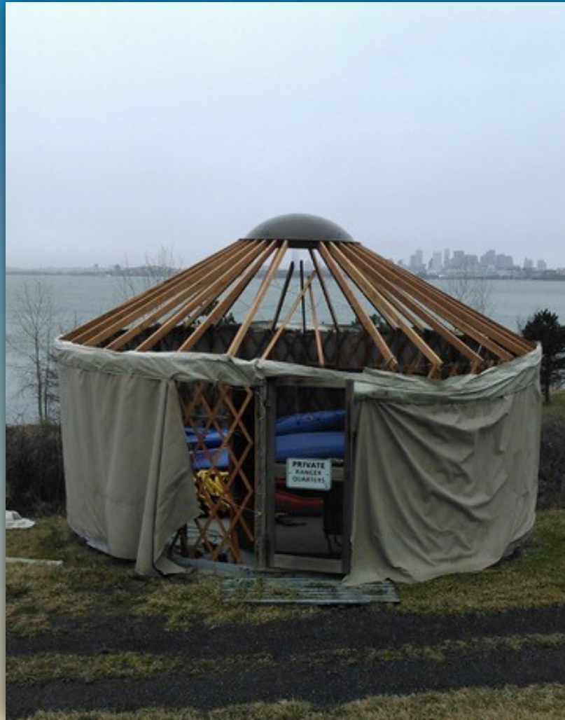
Damage to yurt
