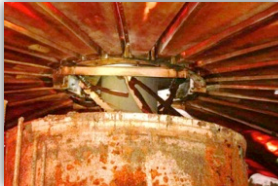
GT 5 & 6: Damaged Center Cage
