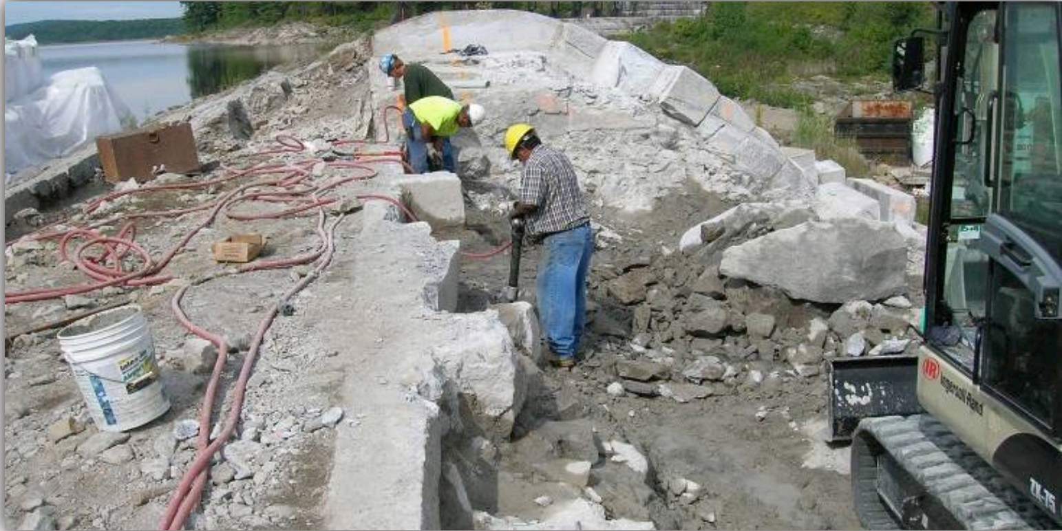
Wachusett Spillway capacity increased by lowering it 2 feet
