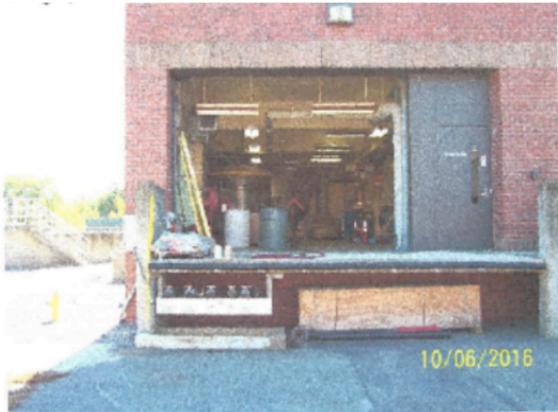
Chemical Building fill station at the north wall
