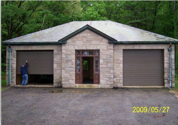
Quabbin Aqueduct Shaft 12 Service Building
