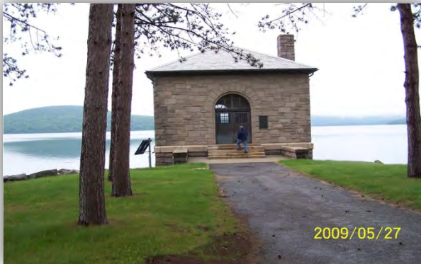
Quabbin Aqueduct Shaft 12 Intake Building
