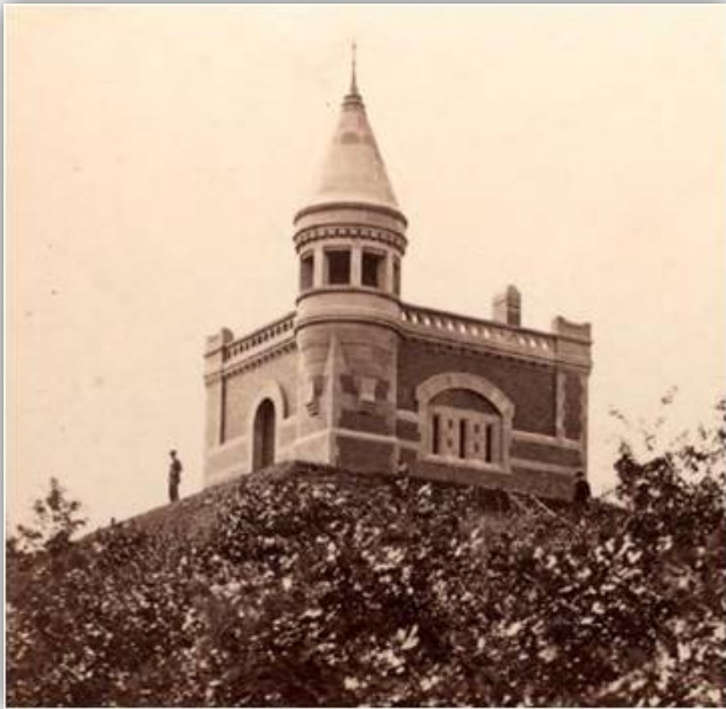
West Siphon Building
