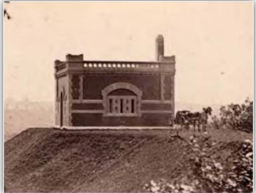
East Siphon Building
