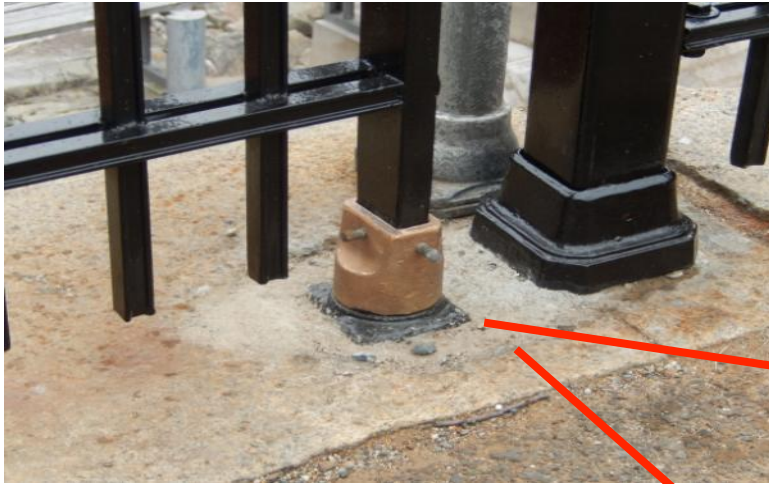
Restored brass gate hardware
