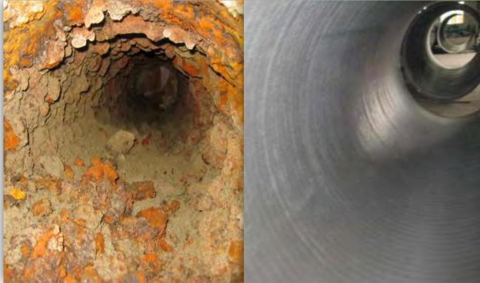
Old unlined cast iron pipe needs to be replaced or cleaned and lined to prevent tuberculation (rust build up), loss of disinfectant residual and potential bacteria growth
