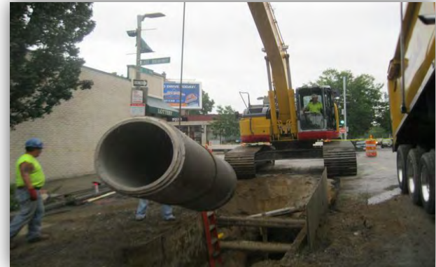
Installation of 30-inch drain on I Street
