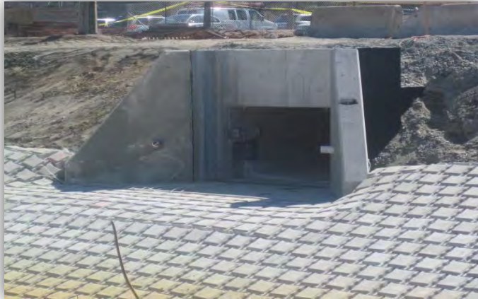
4-ft by 8-ft Stormwater Conduit Outfall
