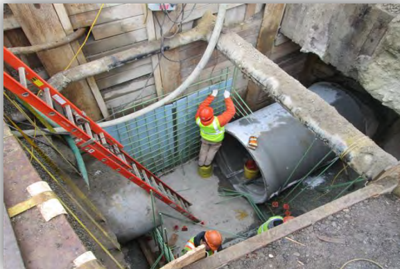
Construction of drain manhole at K and E. 2 nd streets
