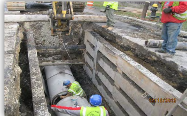
Installation of 36-inch drain on E Street
