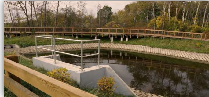
Stormwater Outfall to the Forebay
