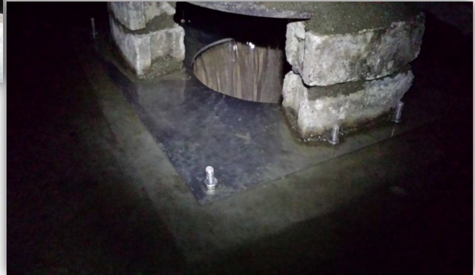
Modified connection to MWRA interceptor
