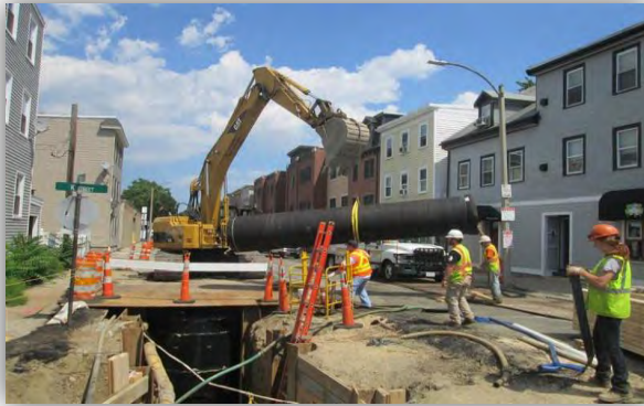
Installation of 42-inch drain on East Second Street
