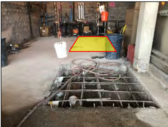
New and existing duct floor penetrations
