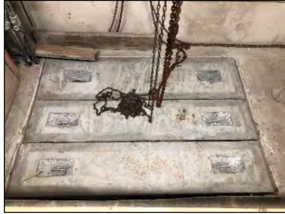
Stainless steel plates to replace concrete planks
