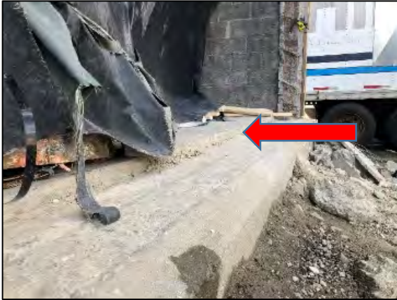
Topping Slab at Grit Bin Room
