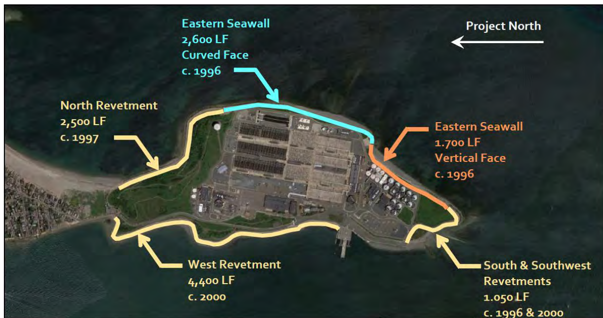
Deer Island Shoreline Protection System
