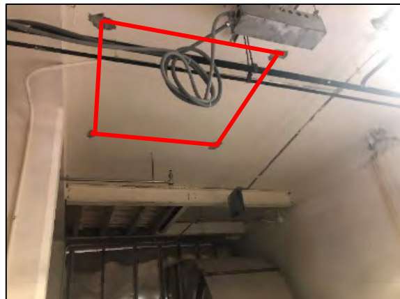
Structural framing required for new penetration
