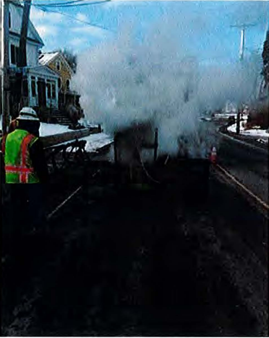
Typical Sewer Lining
