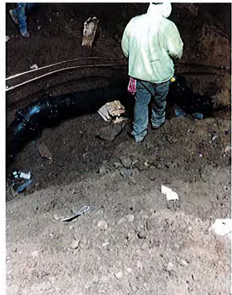
Relocated water lines on Walnut Street at Commerce Way
