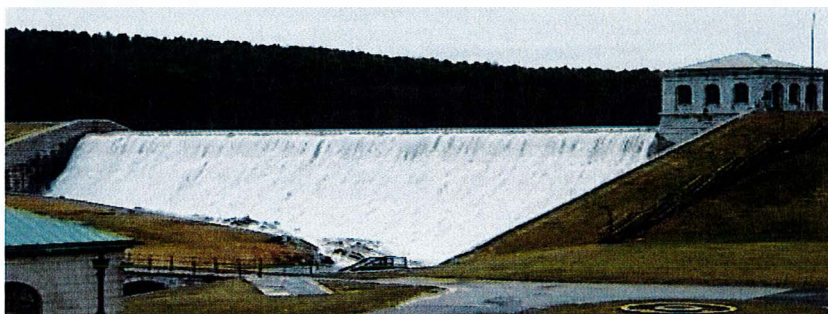
Figure 1 - Sudbury Dam Spillway)
