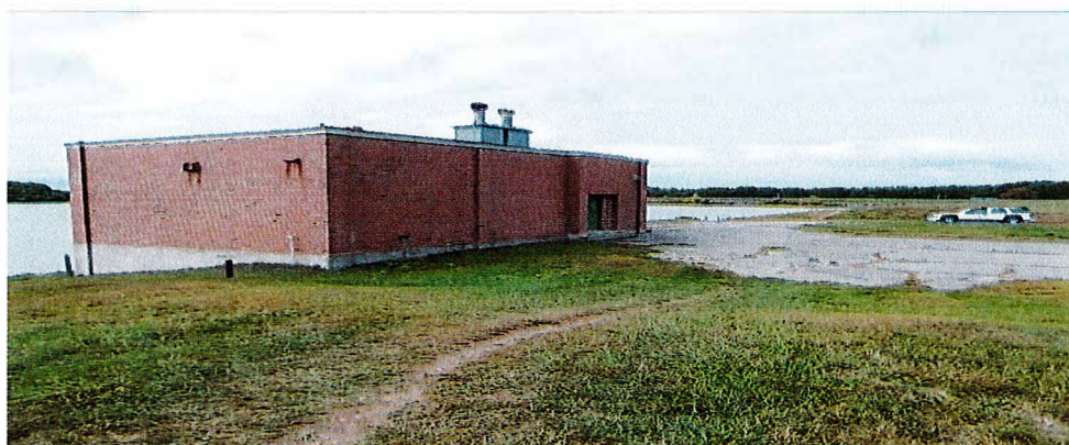
Figure 2 - Leominster Pump Station in notch cut from North Dike
