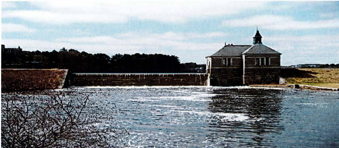
Figure 4 - Foss Reservoir Dam and Spillway
